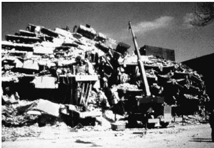
Figura 23 – Colapso total del Hospital Juárez
